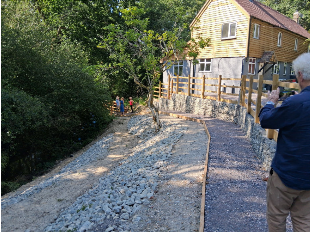
The new approach to the bridge
